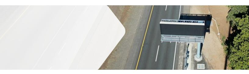
The Front Access Sign by SWARCO Signs has a specific focus on being accessible from the front for upkeep and repairs, which simplifies maintenance procedures. The front access sign plays a key role in enhancing traffic safety, efficiency, and communication by providing drivers with timely and relevant traffic information.
